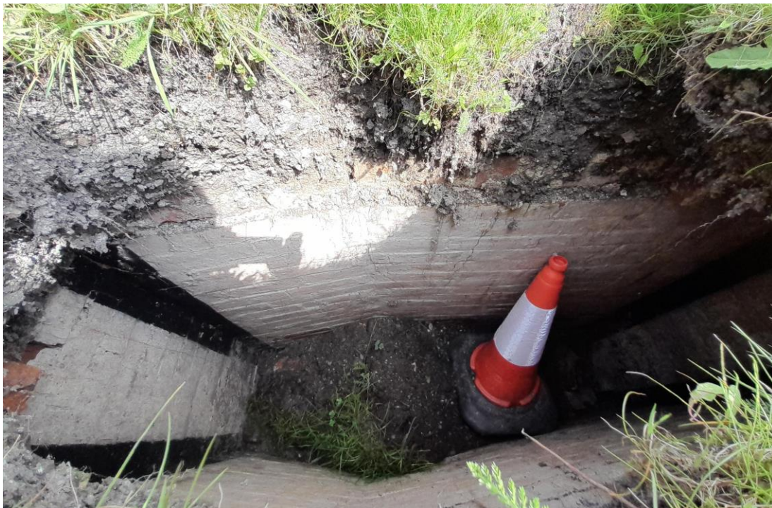
Collapsed brick-lined vault, probably of late 19th-century date, in the graveyard of the Grade I listed Church of St Mary the Virgin, Upavon, Wiltshire. It is unclear if the vault has an occupant below the collapsed material (and traffic cone!). ©Wiltshire Council.
